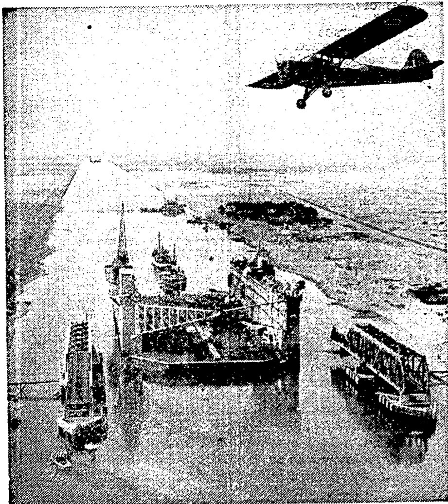
A dock built by the British in Bombay intended for the use of the Royal Navy in Malta, was recently towed there by Admiralty tugs. It is so large (it can accommodate a 50,000 ton ship) that it had to be cut in two for passage through the Suez Canal. This picture shows the first half of the dock being warped through the El Ferdan swing bridge while a RAF spotter aircraft flies over the top. The second half of the dock can be seen approaching up the Canal in the distance.
