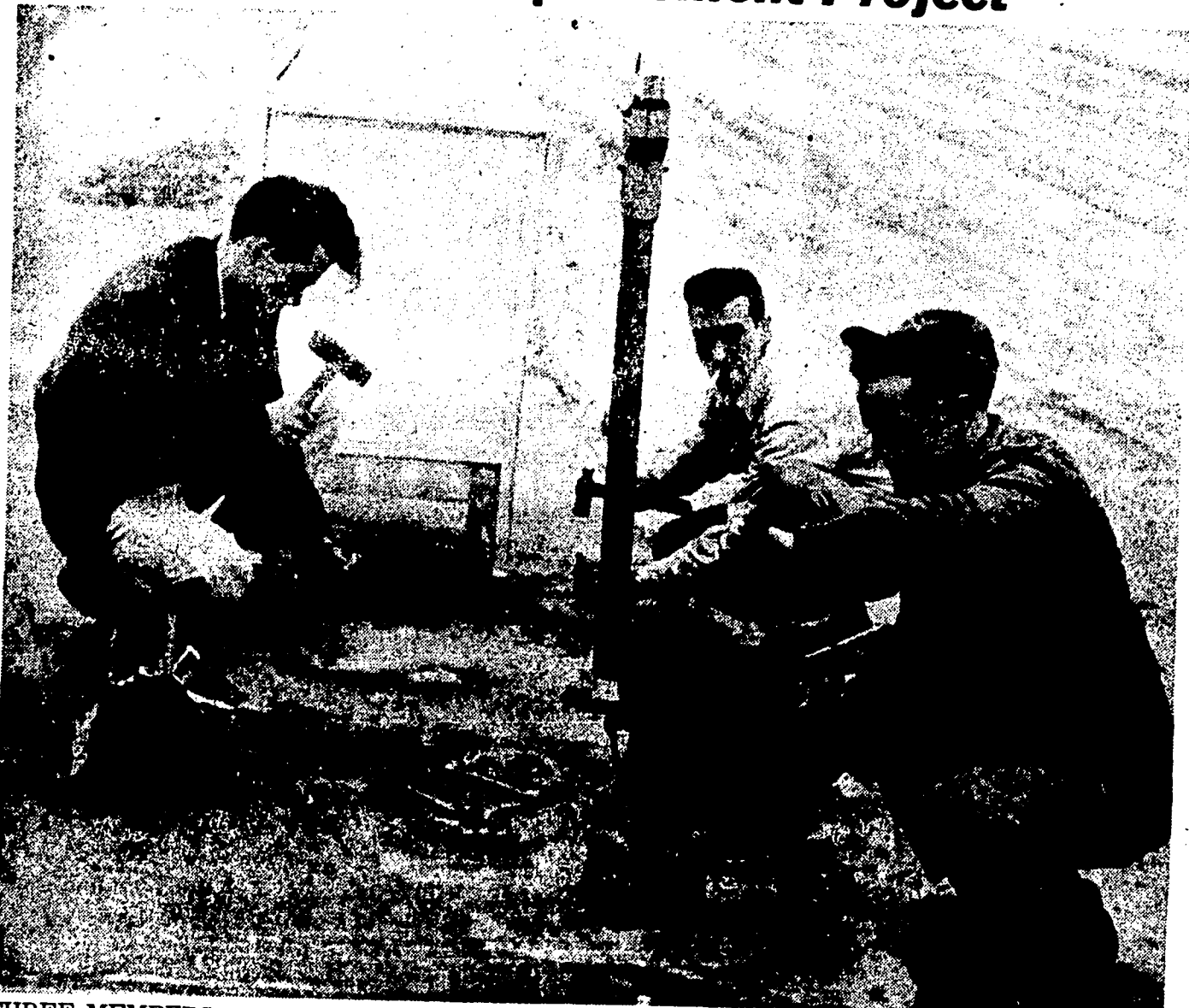
THREE MEMBERS of the Quesnel Jaycees are seen above drilling holes to anchor down the
